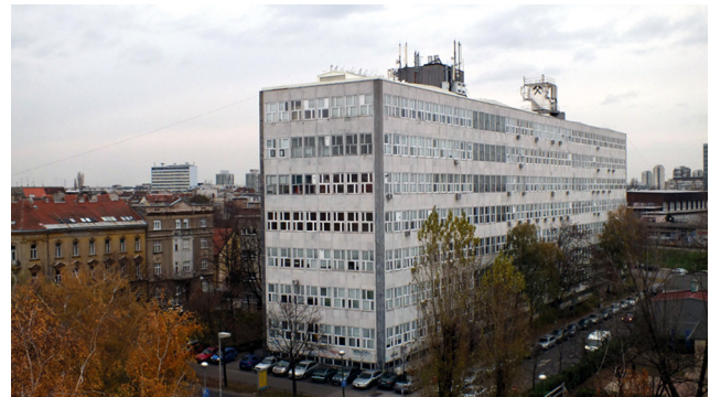
Fig. 6. View of Large Building's north-western façade (present situation)
