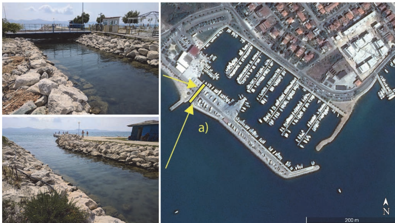
Figure 6. Small craft harbour Vitrenjak in Zadar; a) channel culvert - A = 4 \text{ m}^2
