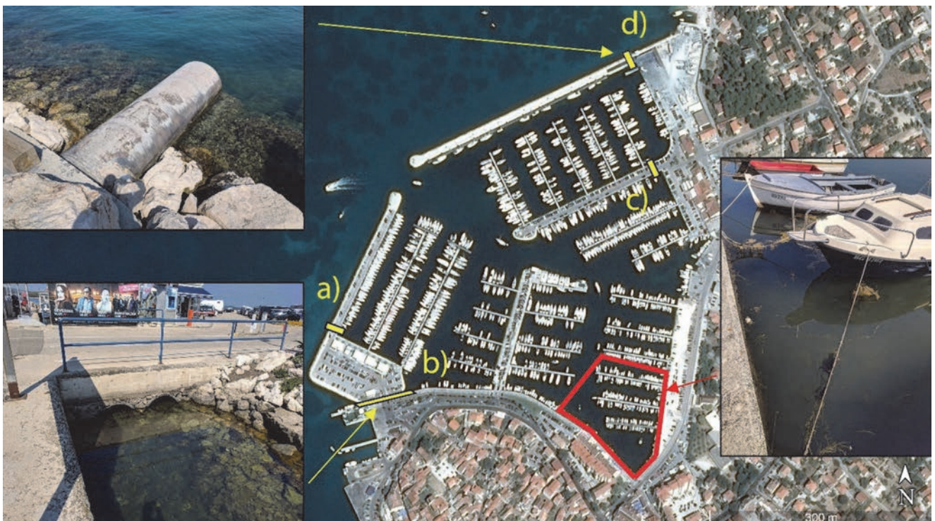
Figure 5. Kornati Marina and small craft harbour in Biograd; a) circular culvert - A = 0,5 \text{ m}^2 ; b) circular culvert - A = 1 \text{ m}^2 ; c) circular culvert - A = 3,6 \text{ m}^2 ; d) circular culvert - A = 1,2 \text{ m}^2 ; dead zone - red polygon
