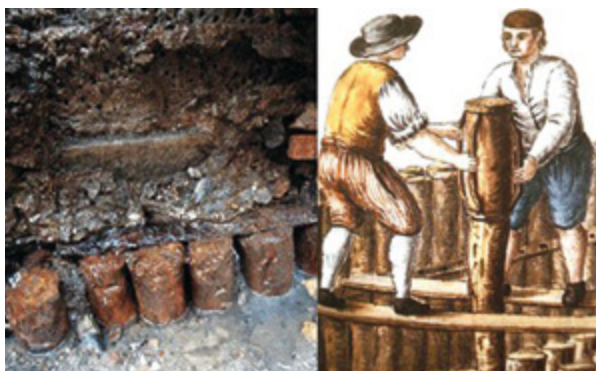
11. Drveni piloti i njihovo postavljanje u Veneciji, URL = http://www.ancient-origins.net/ancient-places-europe/construction-venice-floating-city-001750 (20. rujna 2017.) Wooden foundation beams and their mounting in Venice , URL = http://www.ancient-origins.net/ancient-places-europe/construction-venice-floating-city-001750 (20 th September 2017)
