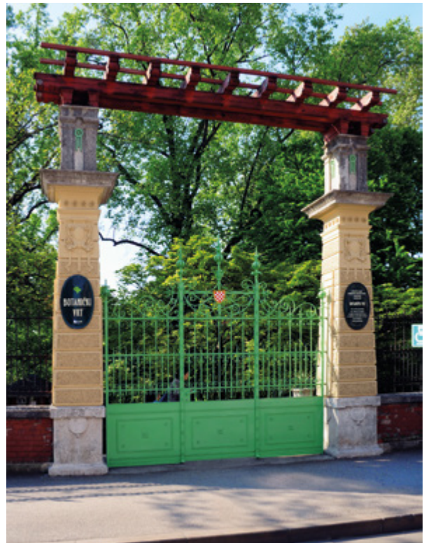
19. Portal glavnog ulaza nakon obnove 2008. (fototeka GZZSKP-a, snimio M. Perušić) Portal of the main entrance after the 2008 reconstruction (GZZSKP Photo Archive, M. Perušić)
