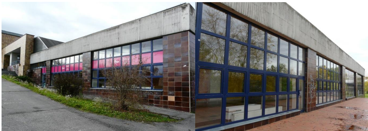
Figure 1. Fenestration of the surveyed structure.
