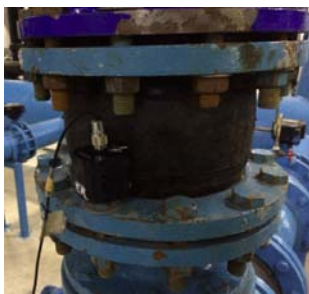
Figure 3. Stretched single ball rubber isolator.
