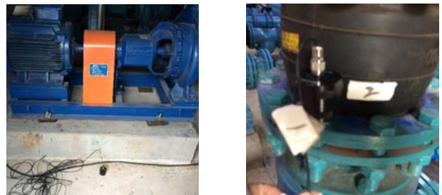
Figure 5. Site vibration test.
