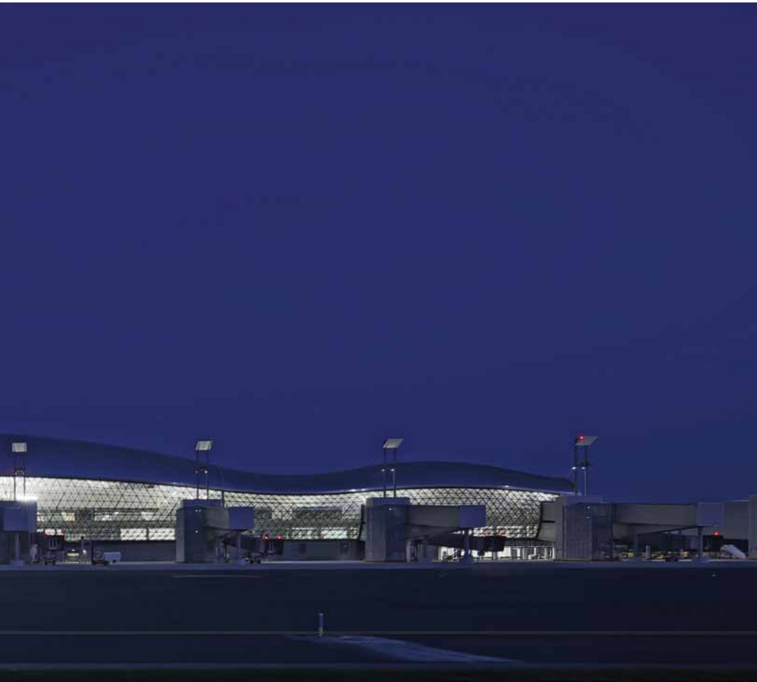
New Passenger Terminal at Franjo Tuđman International Airport Zagreb, exterior 2; author: Damir Fabijanić
