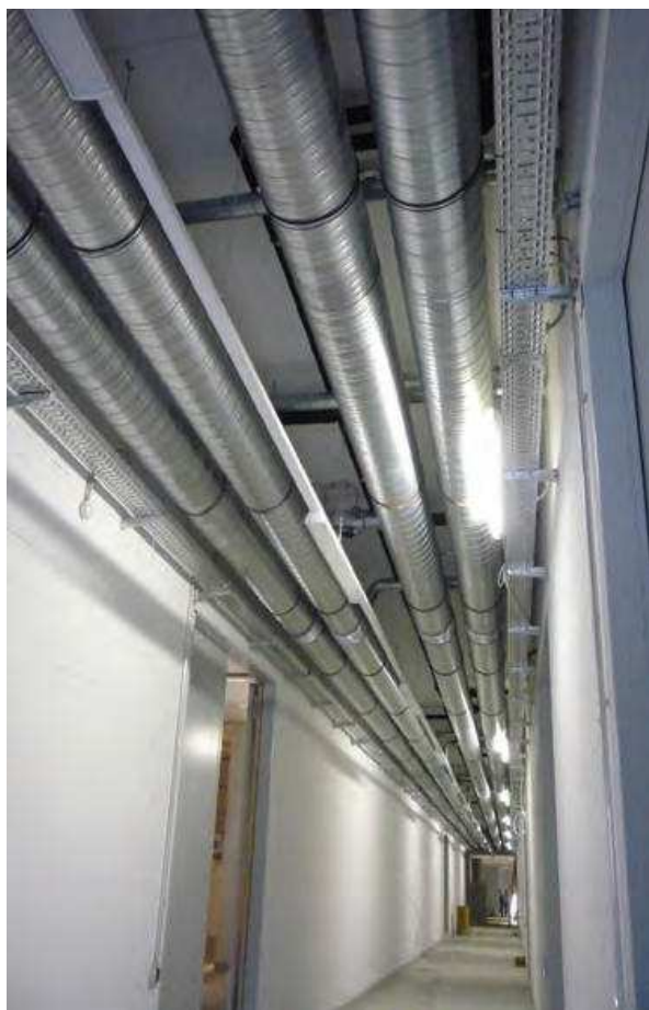
Figure 4. Floor of the Central Art Depot with wiring
