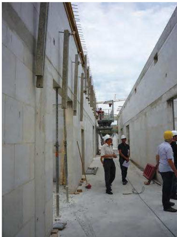
Figure 5. Freiburg storage building during the construction period
