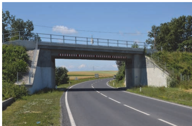
Figure 3. Side view of Weikendorf Bridge in 2016
