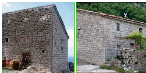
Figure 6 Paštrovska house lean-to roof [12]
