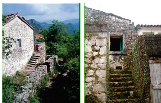
Figure 17 Access to the terrace via an external staircase [26]
