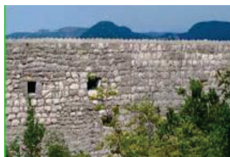
Figure 9 Façade facing the hillside [25]
