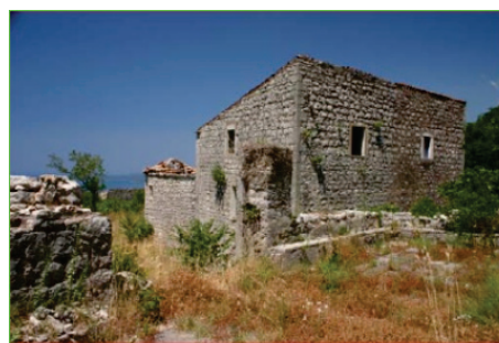
Figure 8 Lateral façade of the row [25]
