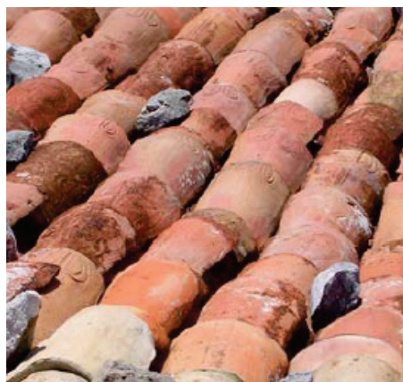
Figure 24 Chute-like tiles, " kanalica " [12]
