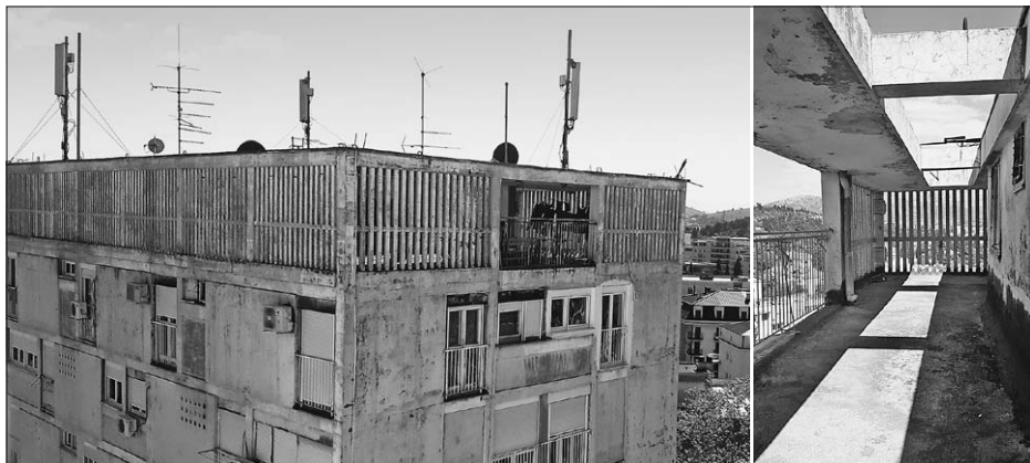
FIG. 14 VERTICAL BRISE-SOLEILS ON THE ROOFTOP TERRACES – A DETAIL MARKING THE DIFFERENCE BETWEEN THE SKYSCRAPERS IN PODGORICA AND THOSE IN SPLIT. A PHOTO AS OF 2019.
