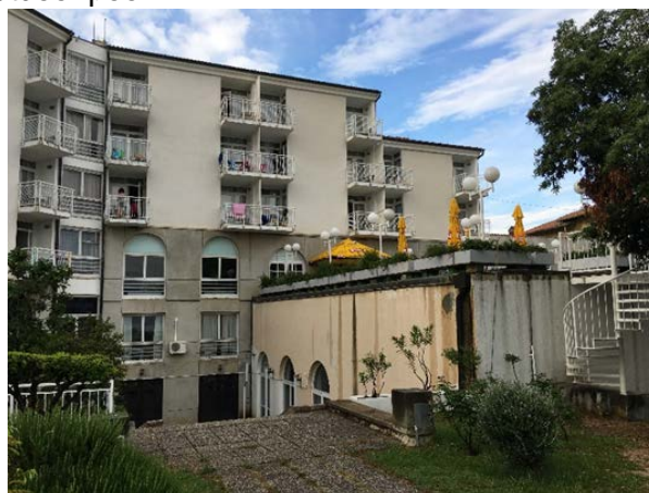
Figure 6. The added building B before the last reconstruction in 2018. Author.
