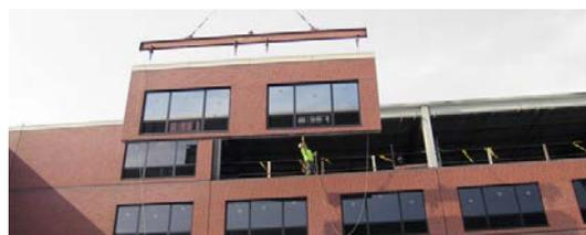
Figure 11. Prefabricated system of brick products [18]
