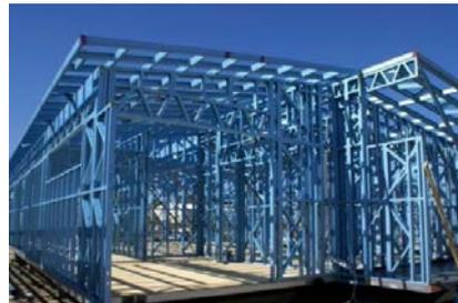
Figure 13. Prefabricated metal system [21]
