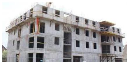
Figure 10. Prefabricated concrete system [17]
