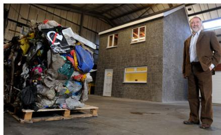
Figure 14. Prefabricated house made of recycled plastics in Great Britain [22]
