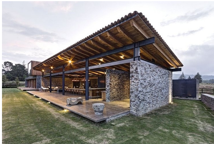
Figure 1. View of the right lamella [14]
