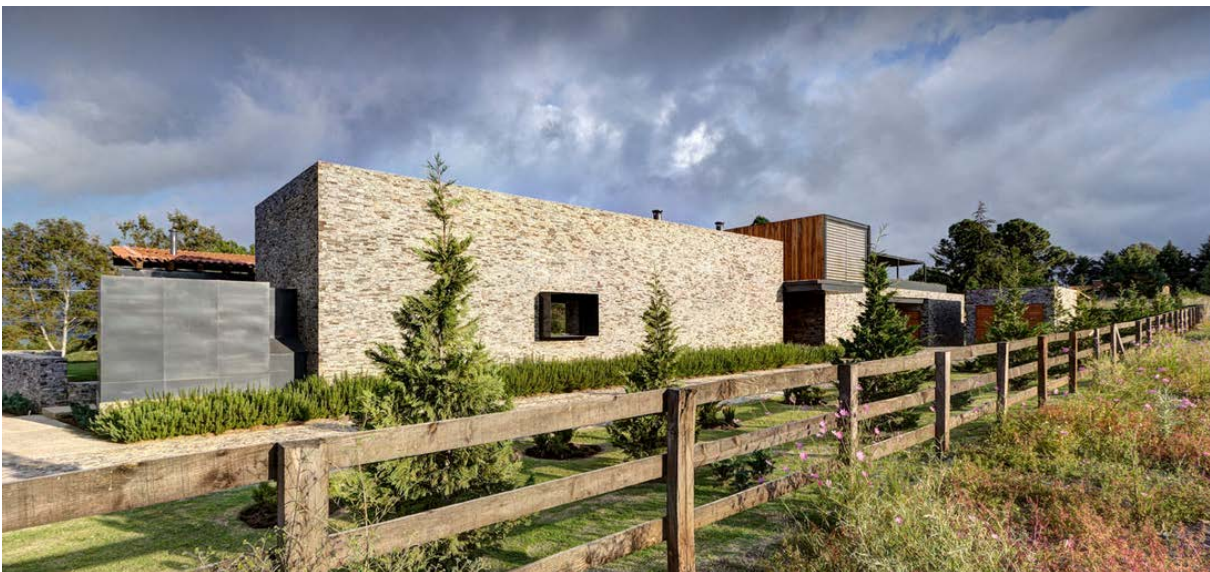
Figure 4. View of the back face [14]
