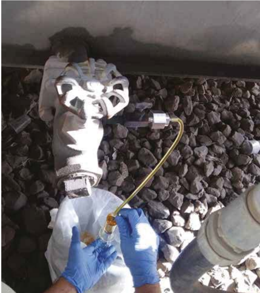
Figure 3. Sampling from the correct valve improves the accuracy of diagnosis
