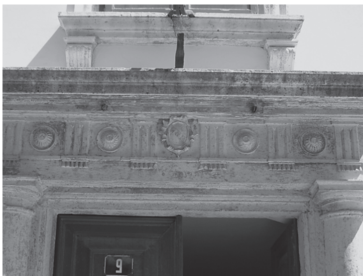
Nadvratnik s trabeacijom na vratima Palače Civalelli u Zadru (foto: P. Vežić) Transom with trabeation on the gate of the Civaleli Palace in Zadar
