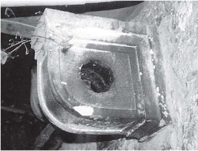
Uho udubljenog profila, zapadno pročelje kuće uz nekadašnji perivoj Cavetto-moulded ear, west façade of the house beside the former park
