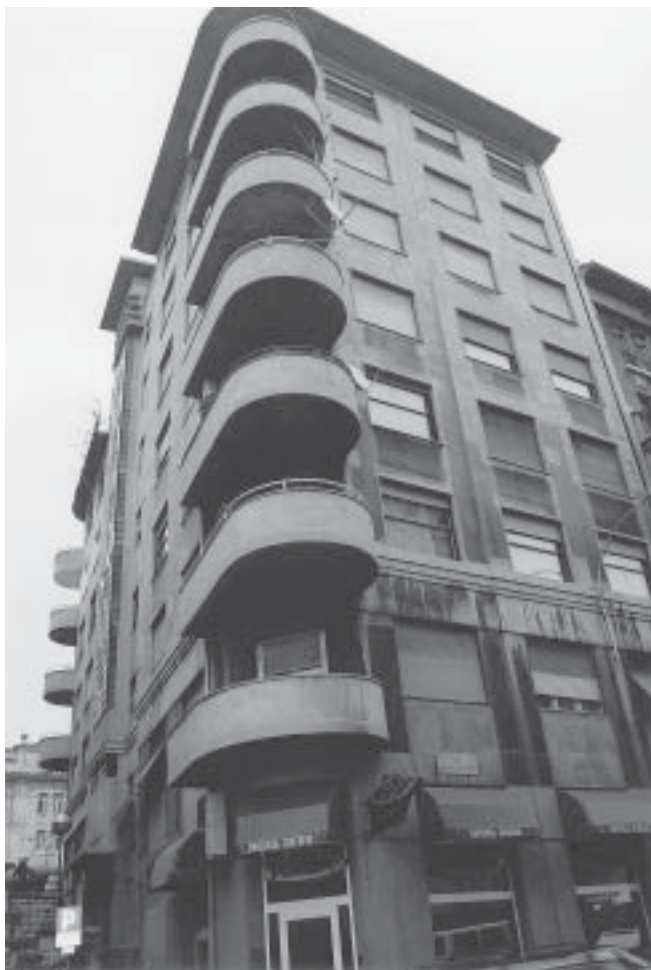
Stambeno-poslovna zgrada u Ulici Blaža Polića 12, zapadno pročelje i jugozapadni ugao Residential-office building, 12 Blaž Polić Street, west façade and south-west corner
