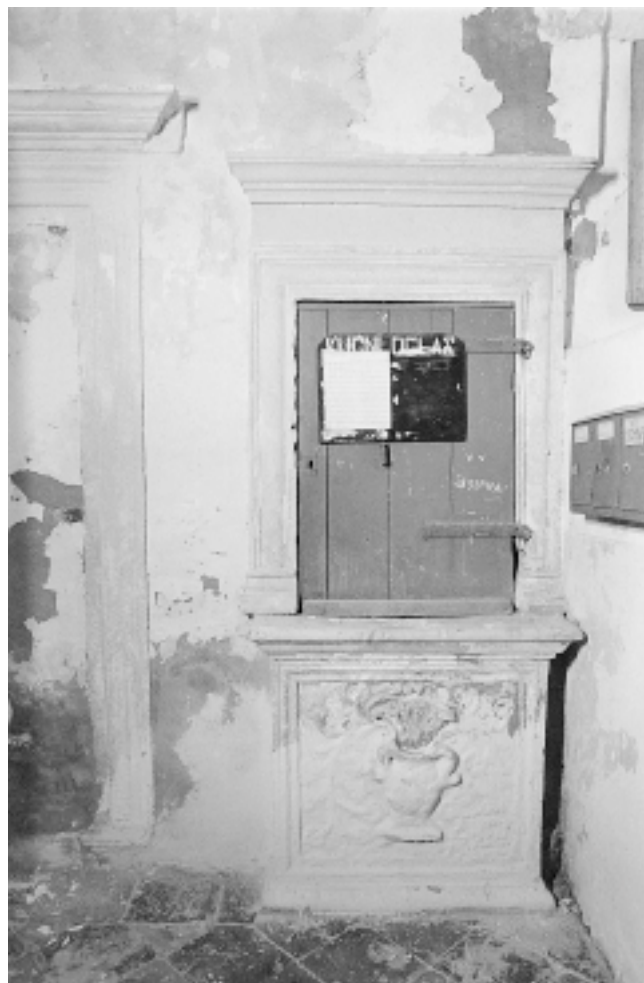
Kruna cisterne u predvorju Entrance hall, cistern top
