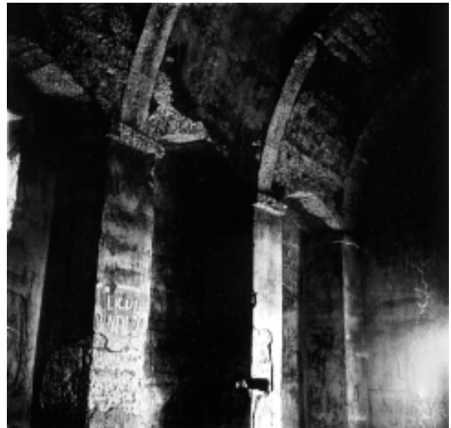
Crkva Sv. Mikule u Dobrovi kod Labina, pojasnice svoda (foto: Državna uprava za zaštitu spomenika kulture i prirode, Rijeka) Church of Saint Nicholas in Dobrova near Labin, reinforced vaults (photo: The State Office for the Protection of the Cultural and Natural Heritage, Rijeka)
