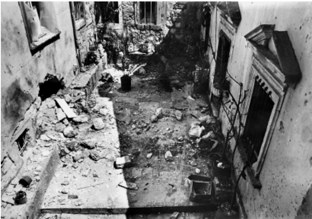
1. Vanjski izgled crkvice nakon granatiranja Dubrovnika 1991. 1. Exterior of the Sigurate church after the shelling of Dubrovnik in 1991
