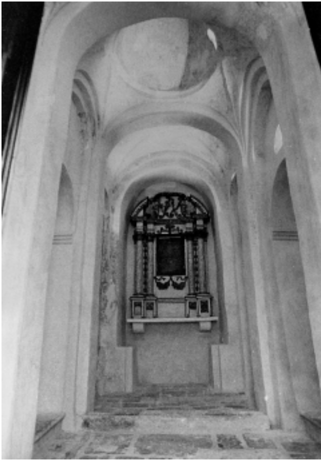
7. Pogled u glavnu lađu nakon obnove 7. View of nave after restoration
