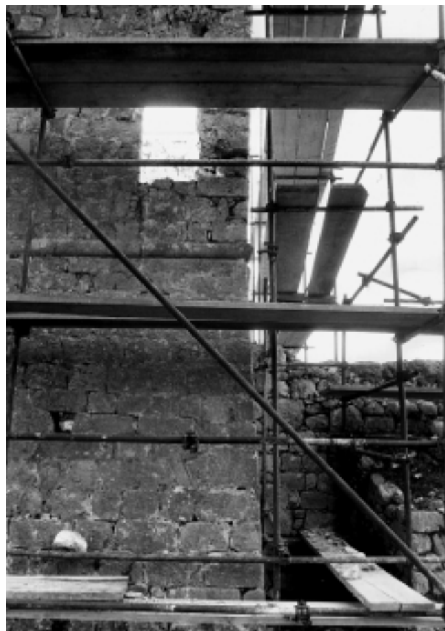
Governor's house, northern facade with slanting bastion wall on the ground floor, rounded cornice, and entrance to destroyed corner sentry box opened during restoration research (photo K. Horvat-Levaj)
