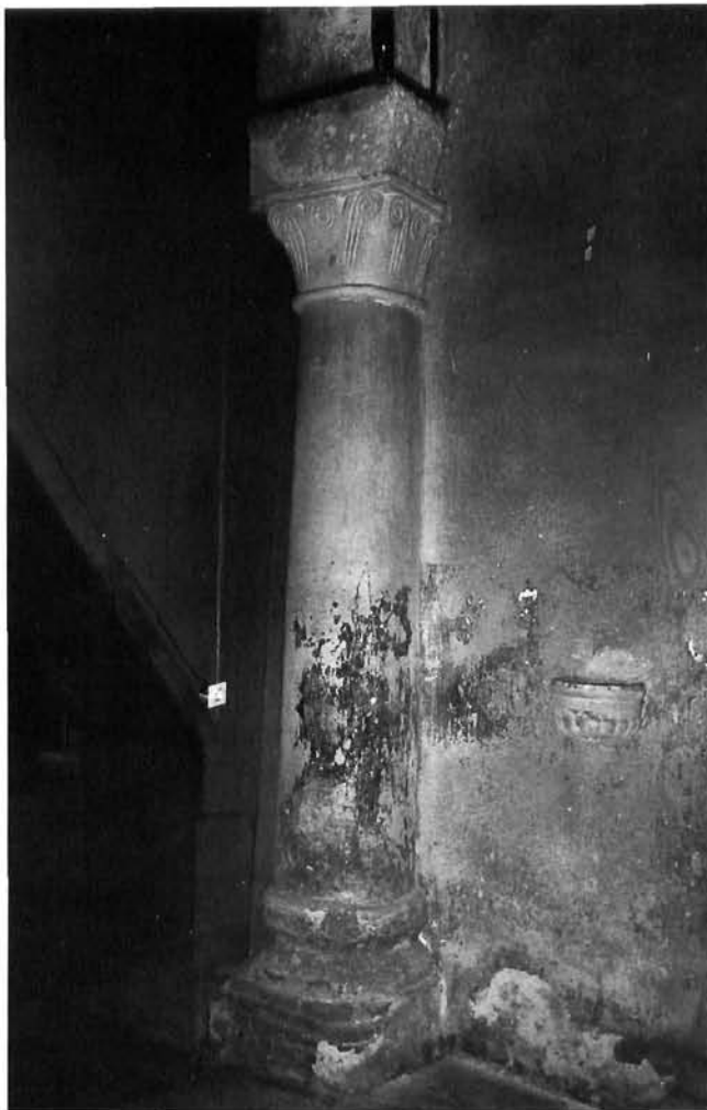
4. Crkva Sv. Martina, sjeverne arkade – polustup prizidan uz pročelje 4. Church of Saint Martin, north arcades - half-column attached to facade
