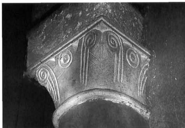
5. Crkva Sv. Martina, sjeverne arkade – impost-kapitel polustupa 5. Church of Saint Martin, north arcades, half-column capital with family insignia
