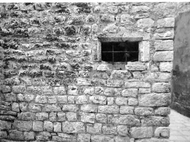
Renesansna gradska kuća, dio sjeverne fasade s karakterističnom strukturom zida i gotičkim prozorom A Renaissance city house, part of the north facade with characteristic wall structure and a Gothic window
