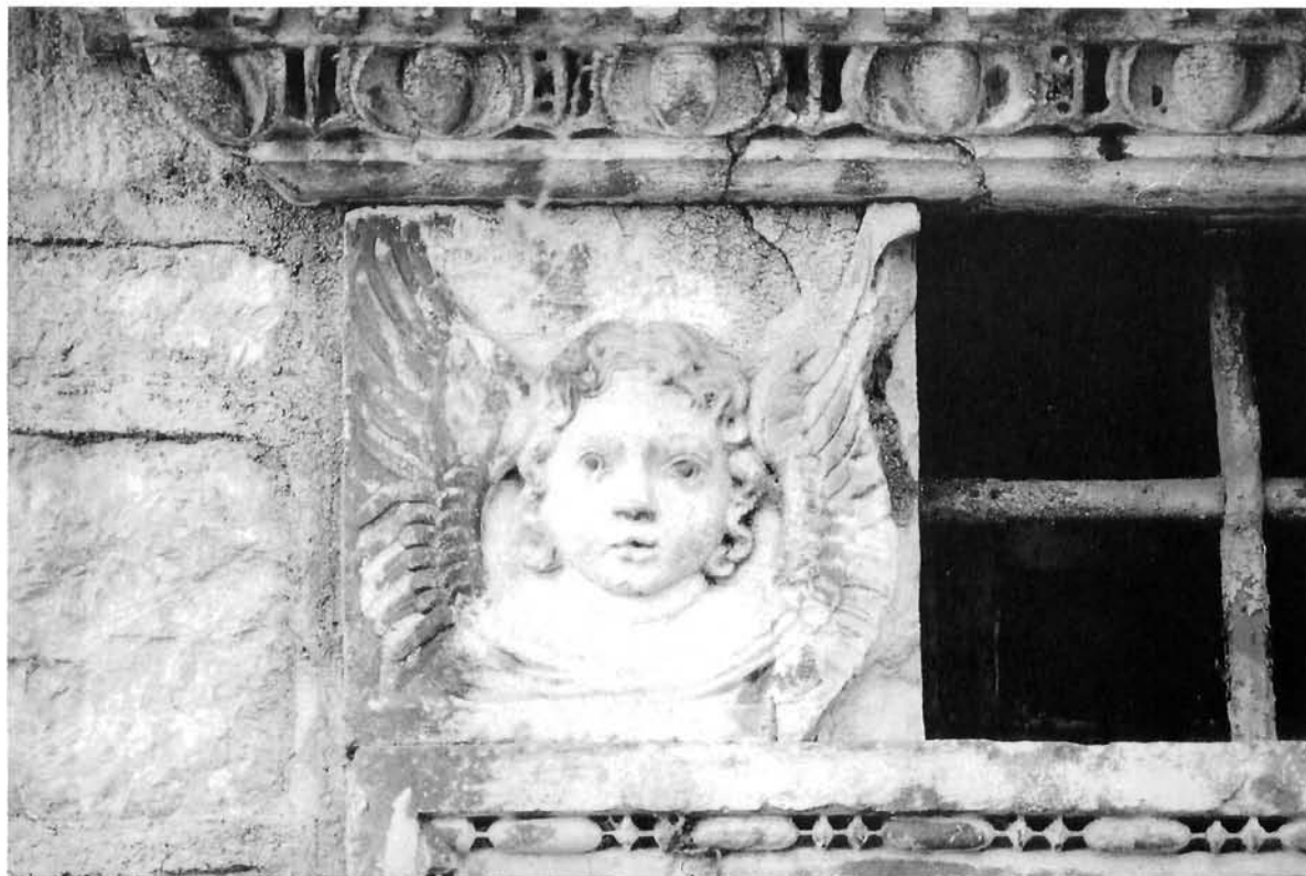
Palača Draganić, detalj anđela s portala na zapadnoj fasadi Draganić Palace, an angel, detail from the west facade portal
