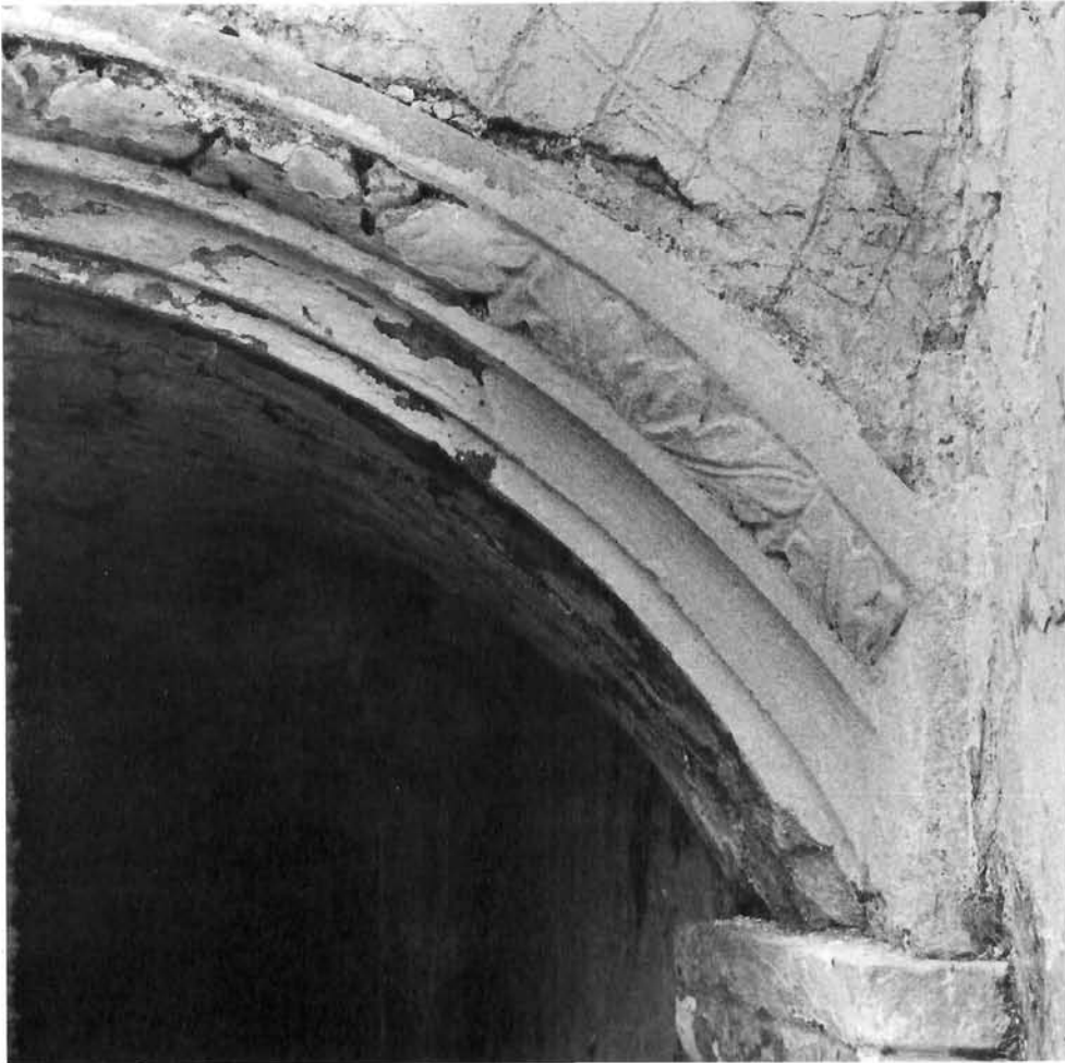
Luk stubišta The arch of the staircase
