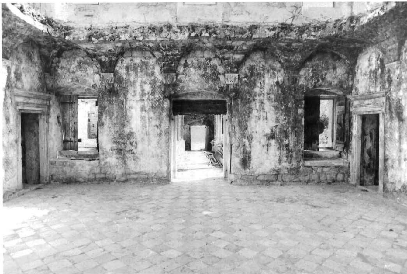
Dvorana prizemlja (saloča), pročelni zid Ground floor hall ('saloča'), front wall
