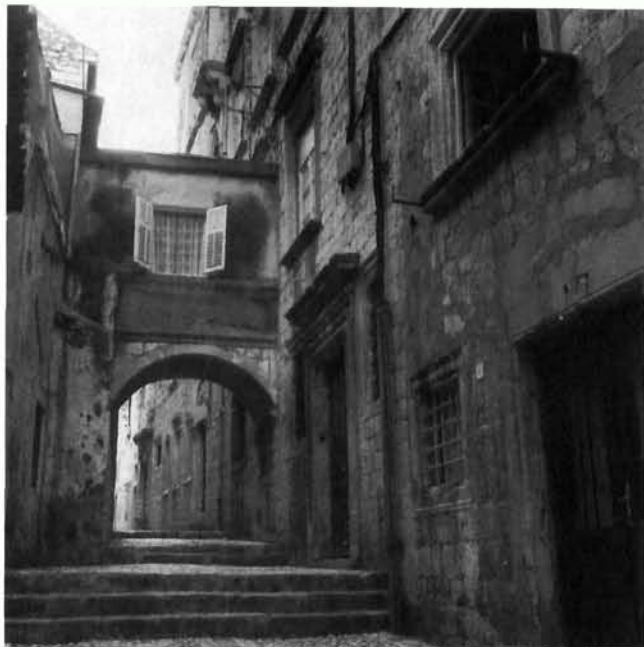
Dubrovnik, most (s recentno nadzidanom prostorijom) koji povezuje kuću iz Andrijićeve ulice br. 8 s terasom (foto: V. Marković) Dubrovnik, the bridge (with a recently built room) which connects the house in Andrijićeva ulica no. 8 with a terrace (Photo V. Marković)
