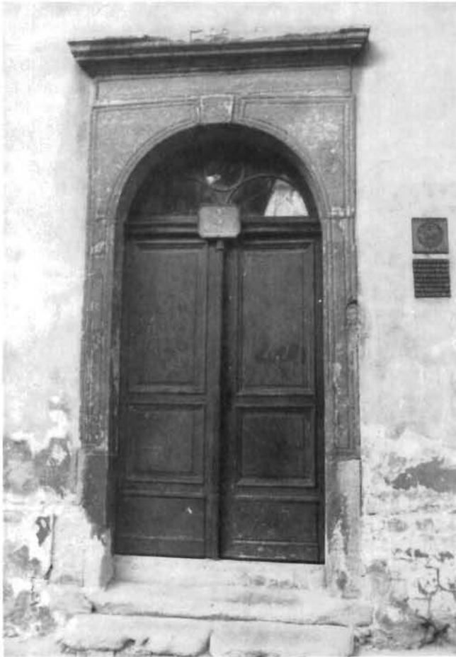
Zagreb, Gornji grad, palača Zrinski, sredina 17. st; portal glavnog (južnog) pročelja palače oblikovan je u kamenu i usklađen s dekoracijom prozora (foto: Mario Krištofić) Zagreb, Upper Town, the Zrinski Palace, mid-17th century; the portal of the main (south) palace facade was formed out of stone and coordinated with the window decoration (photo: Mario Krištofić)
