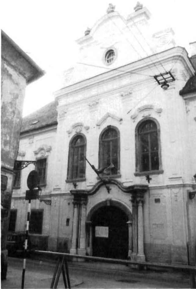
Zagreb, Gornji grad, palača Vojković-Oršić-Rauch, 1764, Matoševa 9; rizalit pročelja kao i ostatak glavne fasade nastao je 1806 (foto: Mario Krištofić) Zagreb, Upper Town, the Vojković-Oršić-Rauch Palace, 1764, Matoševa 9; the projection of the facade as well as the rest of the main facade was made in 1806 (photo: Mario Krištofić)
