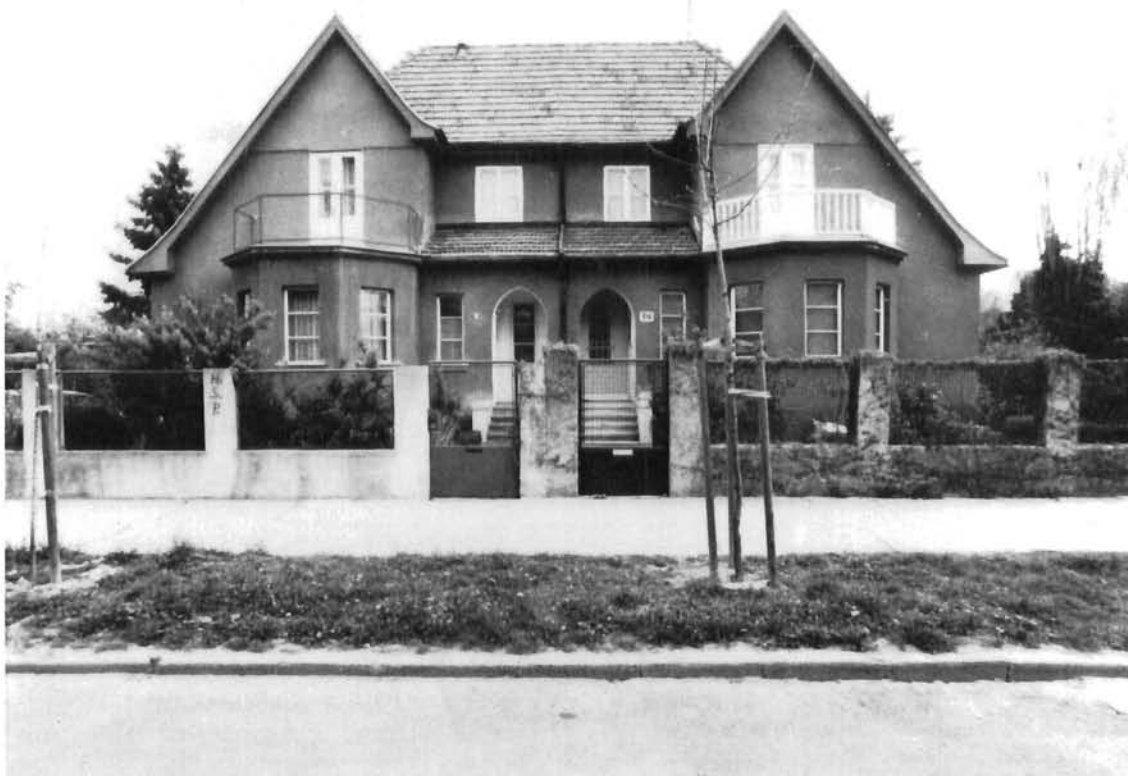
Tipski srodna dvojna obiteljska kuća u Jakićevoj ulici 37–39 u Željezničkoj koloniji (foto: Krešimir Tadić) Double family house of similar type in Jakićeva street 37–39 in the Railroad colony (photo: Krešimir Tadić)
