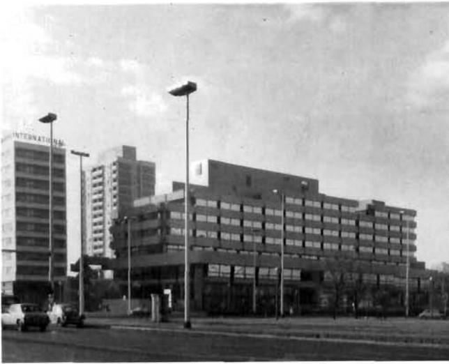
Aleksandar Dragomanović, Radovan Nikšić – poslovna zgrada SDK, Avenija Vukovar 72 (1969-1981) – sjeverno pročelje Aleksandar Dragomanović, Radovan Nikšić – the SDK (Social Accountancy Service) building, Avenija Vukovar 72 (1969-1981) – the north facade
