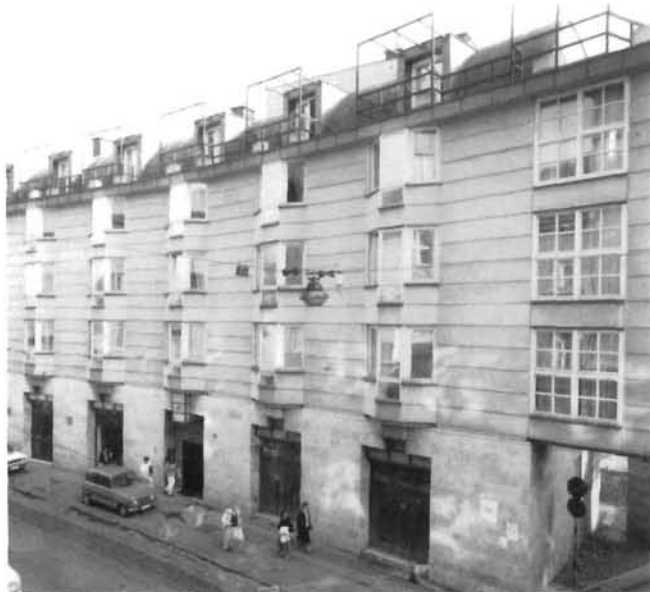
Radovan Tajder – stambeno-poslovna zgrada, Ilica 81 (1984-1986) – ulično pročelje Radovan Tajder – apartment-business building, Ilica 81 (1984-1986) – the street facade
