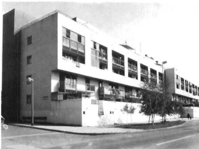
Branko Kincl – stambena zgrada u naselju Klaka, Grižanska ulica (1978-1981) – zapadno pročelje Branko Kincl – apartment building in residential quarter Klaka, Grižanska street (1978-1981) – the west facade
