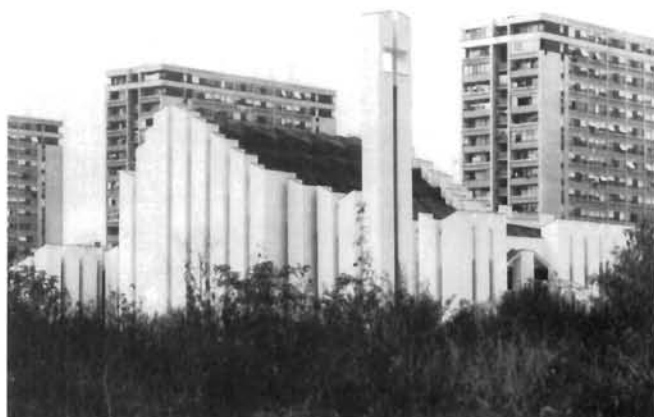
Matija Salaj, Egon Seršić – crkva sv. Križa na Sigetu (1973-1983) – južno pročelje Matija Salaj, Egon Seršić – Church of the Holy Cross in Siget (1973-1983) – the south facade
