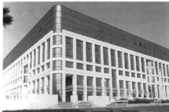
Velimir Neidhardt – poslovna zgrada INA – Trgovina, Avenija V. Holjeveca (1986-1988) – pročelje Velimir Neidhardt – the INA Trade building, Avenija V. Holjeveca (1986-1988) – the facade
