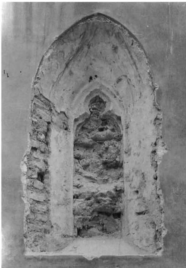
Crkva sv. Križa, ranogotička monofora broda (otvorena prilikom restauratorskih istraživanja 1988) (foto: Katarina Horvat-Levaj) The church of the Holy Cross, early Gothic monofore of the nave (revealed during restoration investigation in 1988) (Photo Katarina Horvat-Levaj)
