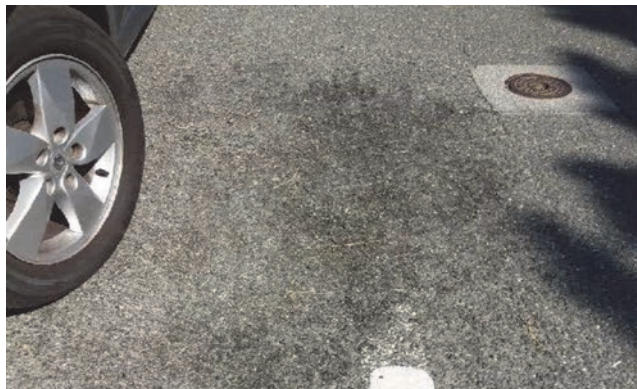
Figure 5. Detail of driving surface wear
