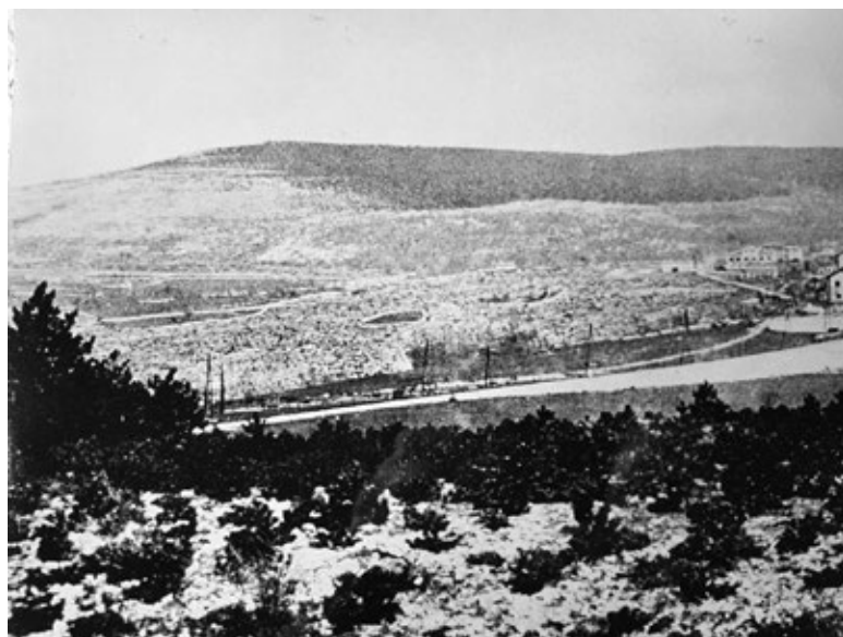
Figure 4 Railroad station Herpelje around 1870 (Source: Department of Forest administration, Postojna)
