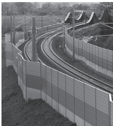
Slika 3. Panelni bukobrani Figure 3. Panel noise barriers
