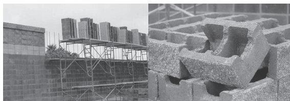
Slika 4. Zidani bukobrani Figure 4. Masonry noise barriers
