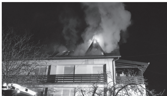
Slika 5. Požar u trenutku kada su ga primijetili ukućani Figure 5. Fire at the moment it was perceived by the persons in the building
