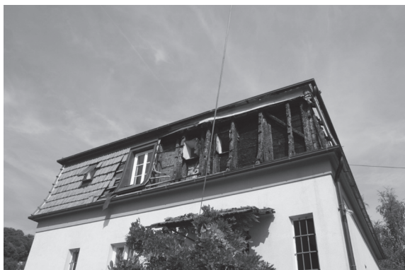
Slika 3. Tragovi požara u potkrovlju stambenog objekta Figure 3. Traces of fire in the attic of a housing building
