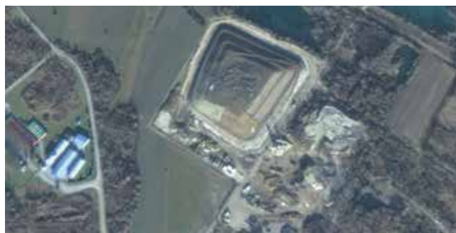
Figure 2. Satellite image of the Trebež waste site during remedial activities (photo taken on 25 December 2015), source: Google Earth
