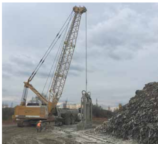
Figure 6. Equipment for excavation of diaphragm, inlet channel and entrance funnel
