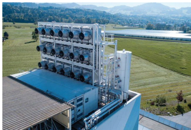
Slika 2 – Climeworksovo postrojenje za hvatanje CO 2 iz zraka (izvor: https://www.euractiv.com/section/climate-strategy-2050/interview/fri-ready-scientist-im-pretty-sure-we-will-need-carbon-removal-technologies/ )
