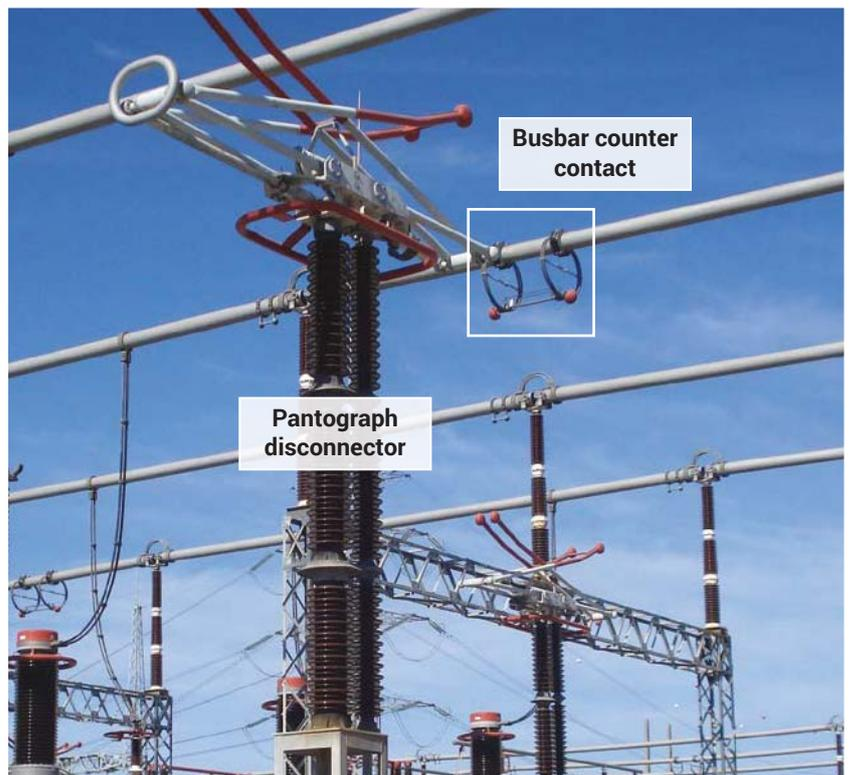
Figure 6. Pantograph disconnectors' busbar counter contact
