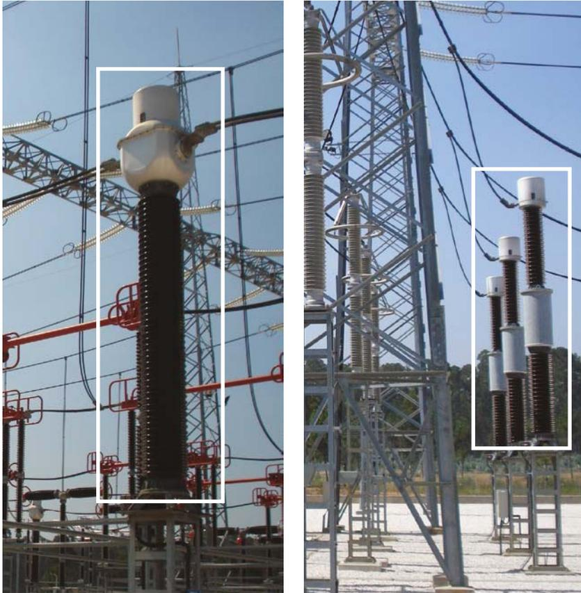
Figure 7a and 7b. Current transformer (left) and voltage transformer (right)
