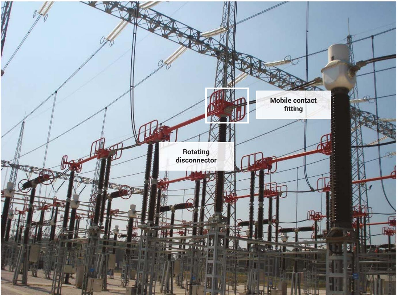
Figure 5. Rotating disconnector fitting
