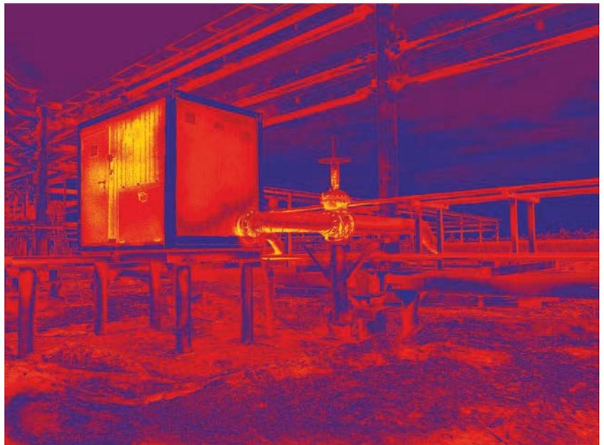
Figure 2. Hotspot detected by infrared thermography
