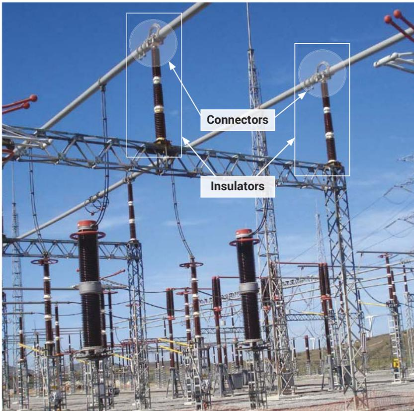
Figure 3. Insulators and connectors for rigid busbar
