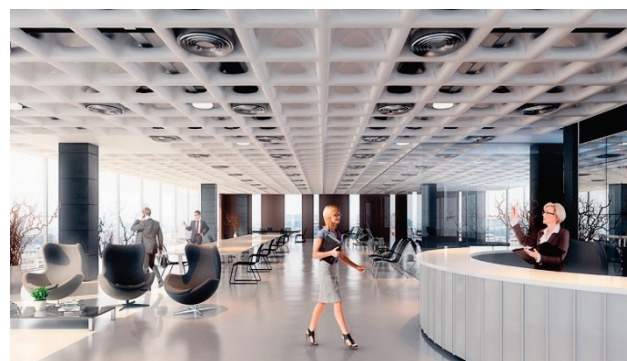
Figure 5 Holedeck two-way waffle RC floor slab as an ideal solution for large spans and therefore adaptable, energy efficient and seismically safe public and residential buildings ( http://holedeck.com/en/edificacion-en-altura )
