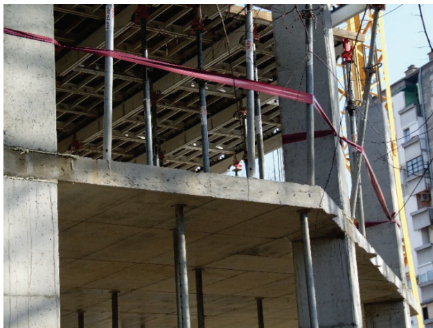
Figure 4 Example of thick and heavy concrete slab (Zrinskog i Frankopana street in Subotica)
