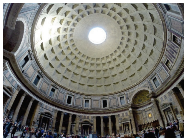
Figure 3 Coffered ceiling of the Roman Pantheon built early in the first millennium ( http://www.monolithic.org/domes-more/the-pantheon-rome-126-ad/photos )
