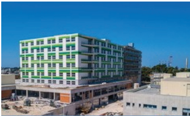
FIGURE 2. The new hospital.
