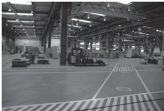
Slika 5. Industrijska hala Figure 5. Industrial plant
