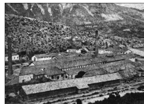
FIG. 3. STEAM-POWERED BRICKYARD BEFORE DEMOLITION, 1919
