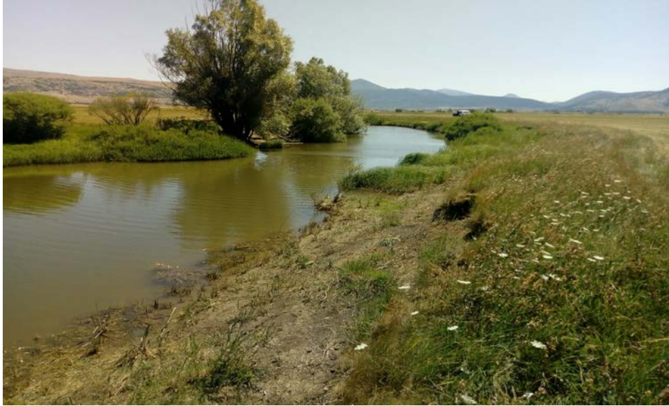
Figure 2. Šuica River bank - existing condition
