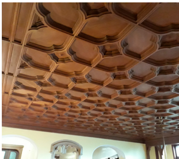
11. Drveni strop u dvorcu Hilleprand-Mailáth u Donjem Miholjcu, 1903. – 1907. (snimio D. Trcović, 2018.) Wooden Ceiling in the Hilleprand-Mailáth Castle in Donji Miholjac, 1903–1907 (D. Trcović, 2018)
