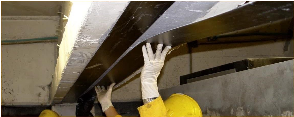
Figure 7 Flexural strengthening (CNR-DT [7])
