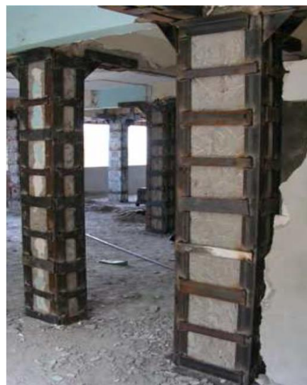
Figure 4 Steel jacketing applied to RC columns (P.Gavrilovic [14])
