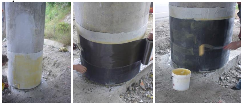
Figure 8 Confinement strengthening (Di Ludovico M [20])
