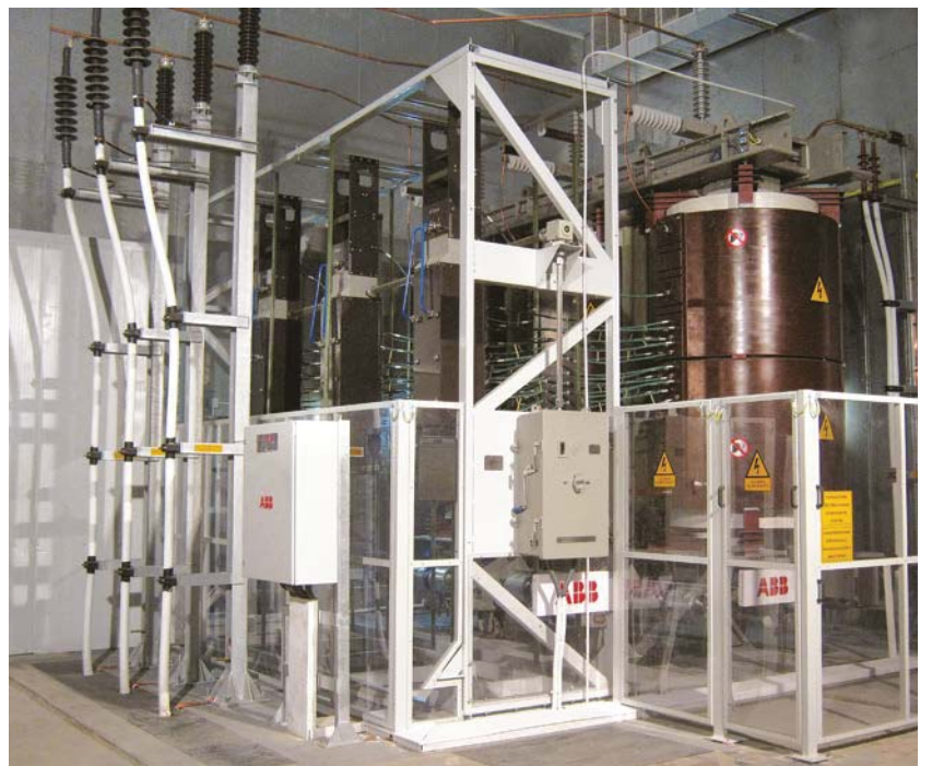
Figure 5. 72 kV HiDry transformer with OLTC
