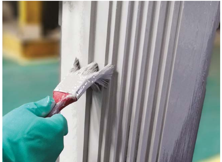
Figure 8. Paint run, sagged or wrinkled paint surface should be evened out with the surrounding surface
