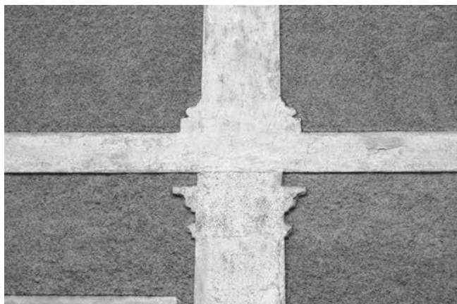
8. Detalj žbukanih pilastara i trake na pročelju, 2013. Detail of the plastered pilasters and strips on the façade, 2013
