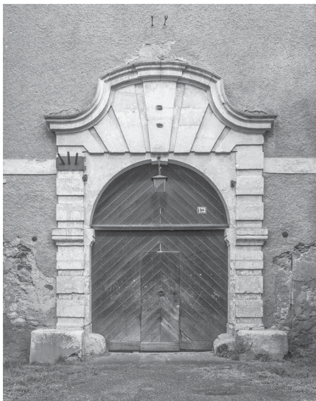
9. Glavni portal, 2019. Main portal, 2019
