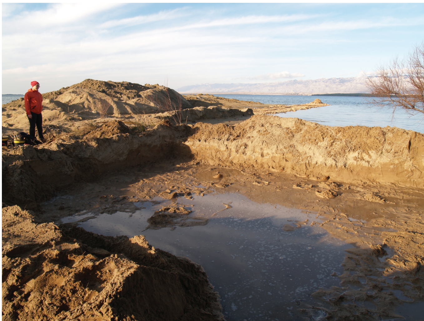
Slika 4. Početak radova Figure 4. Beginning of excavations
