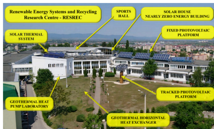
Figure 1. Renewable energy systems installed in the RESREC Research Centre in the Colina Campus of the Transilvania University of Brasov, Romania
