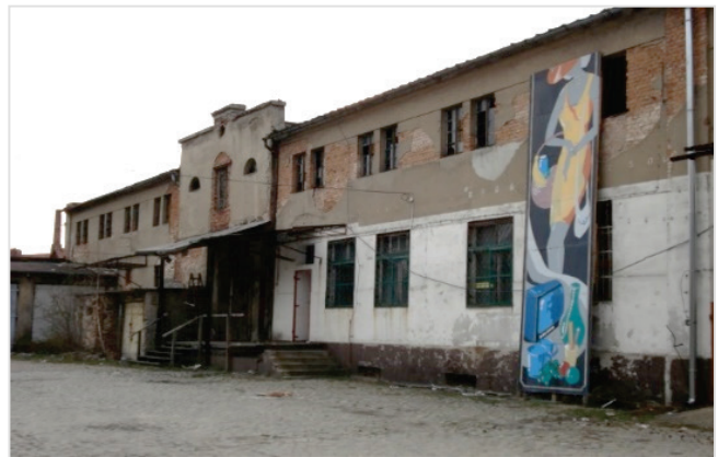
Figure 3 Southeast elevation of building (second part) prior to adaptation
