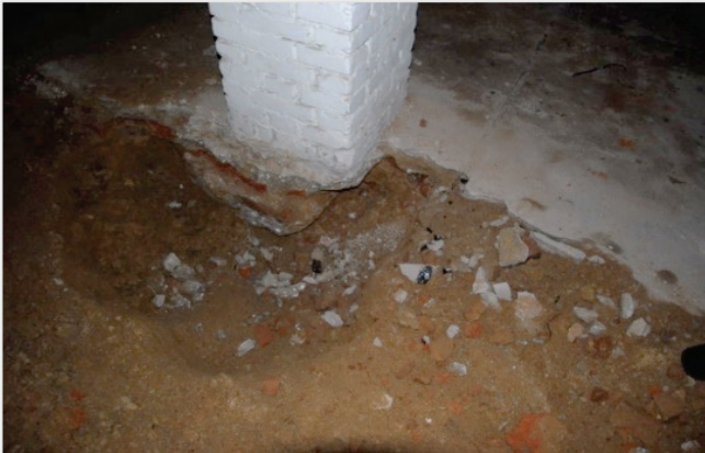
Figure 6 Existing brick foundation footings under some of the posts
