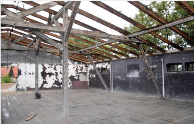
Figure 7 Queen post roof truss structure during renovation works
