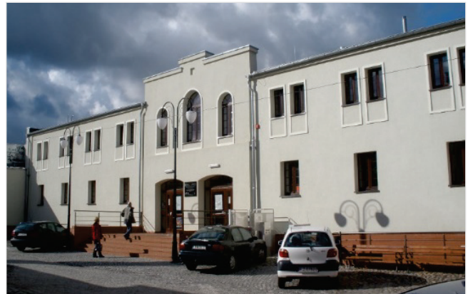
Figure 4 Southeast elevation of building (second part) after adaptation
